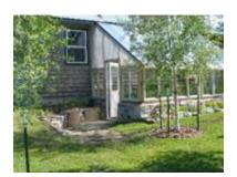
The 10' x 20' greenhouse is a partially below-ground add-on to the house; a stone retaining wall was constructed below the double-pane windows. The sloped roof is triple-wall polycarbonate, which insulates as well as the windows. Doors at each end provide ventilation, as will temperature-activated, louvered polycarbonate panels above the doors.
