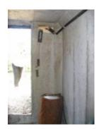
An outer and and inner door provide entrance to the cellar. The floor is dirt; the septic tank cover in the ceiling is sealed shut. A 2" aluminum vent pipe exits through the ceiling and soil cover, and elbows to prevent moisture from getting into the pipe. There is no cold air intake vent; the doors provide sufficient air leakage. Electricity has been added, for light, and also for heat if needed, in the winter. The heater is an old rusty can with a light bulb inside.
